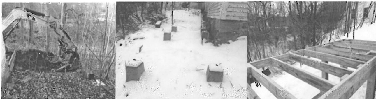
Addition of deck for fire escape
